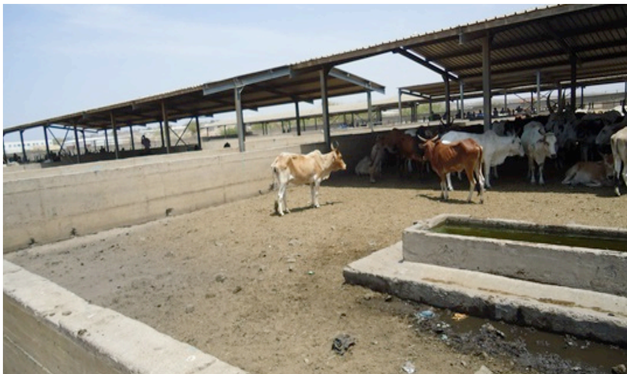
Good marketing infrastructure with sheds for protecting animals, providing feed and water, and separate animals
