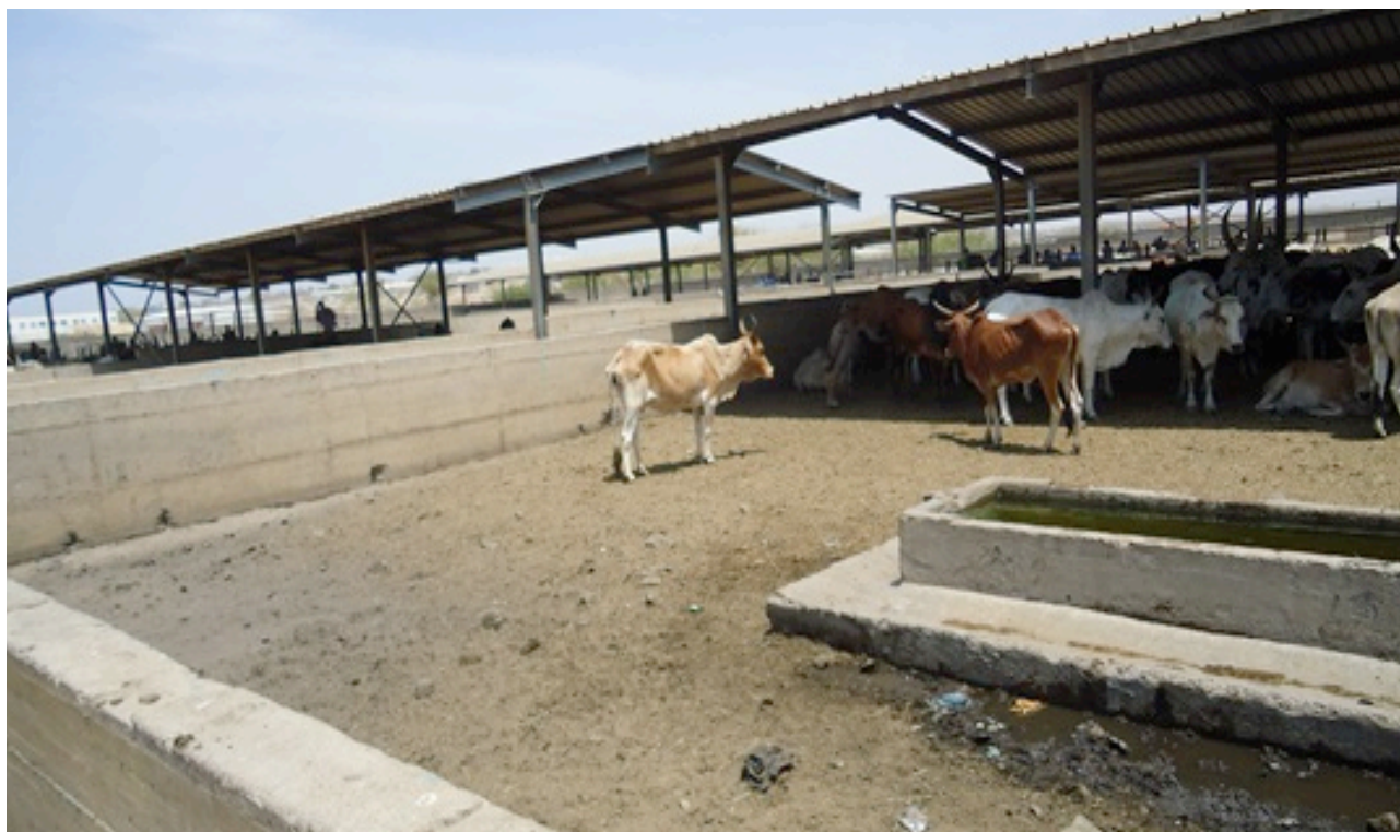
Good marketing infrastructure with sheds for protecting animals, providing feed and water, and separate animals
