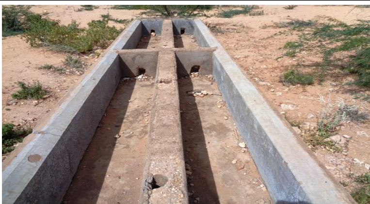
Water trough in poor condition which lack water piping connectivity- Rhamu
