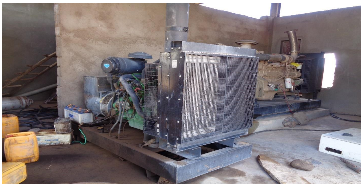
Figure 6 Broken Genset at HallaBorr
