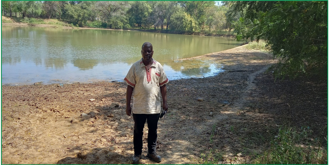
GPS coordinates recorded for a dam in Kurmuk, Assosa
