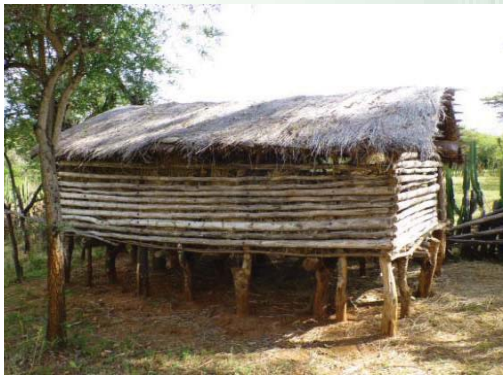
Plate 123: Traditional hay store made using locally available materials
