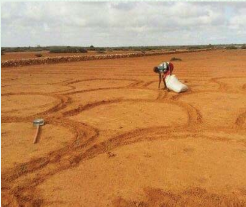
Plate 69: Design of semi-circular bands for water harvesting to support rangeland rehabilitation
