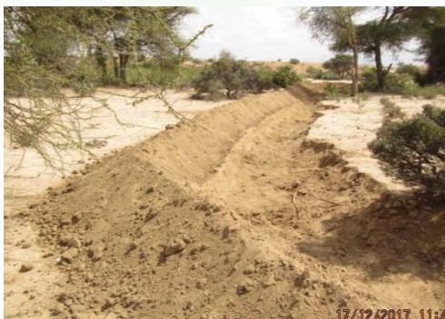
Plate 67: Contour Terracing for rangeland rehabilitation and reseeding
