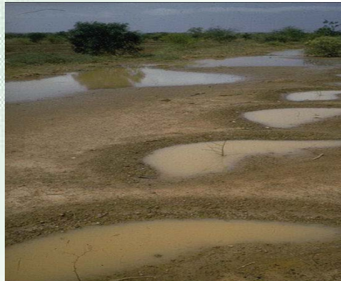
Plate 69: Design of semi-circular bands for water harvesting to support rangeland rehabilitation
