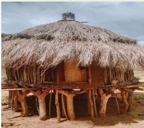
Plate:114: Open and naturally ventilated Traditional seed storage by communities in IGAD region/Karamoja Uganda
