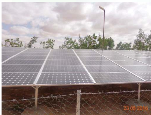
Plate 91: Solar-powered water pump- drawing water from a borehole enough to irrigate fodder. Photo Source FAO Pasture production Manual
