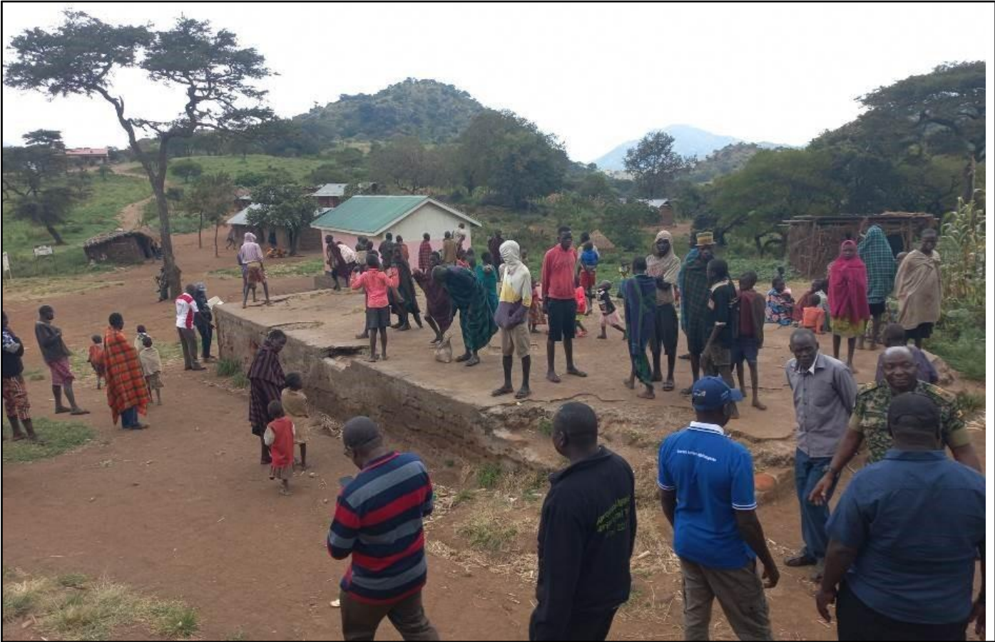
IMAGE OF THE EXISTING DRYING PLATFORM
