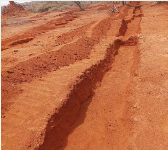
Plate 70: Water Retention ditches developed for reduced runoff and increased soil and water conservation for pasture establishment and rangeland rehabilitation
