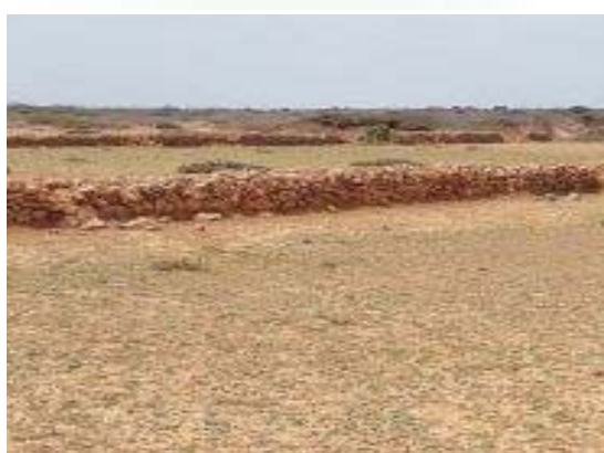
Plate 68: Stone contour placement for increased soil and water conservation in pasture farms.
