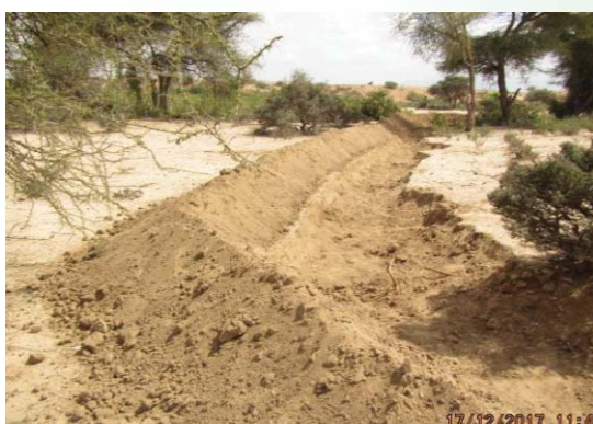
Plate 67: Contour Terracing for rangeland rehabilitation and reseeding
