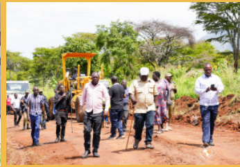
Clearance of the 62Km Usake-NewKuch road in Kaabong, Uganda
