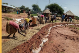
Half-moons construction by Community Members in Rupa, Uganda
